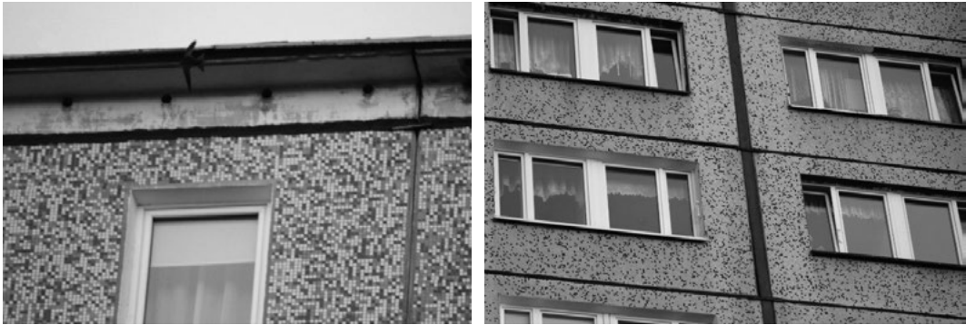
Figure 1. Main places in panel buildings where swifts build nests: ventilation holes in attics (left) and crevices between panels (right)
