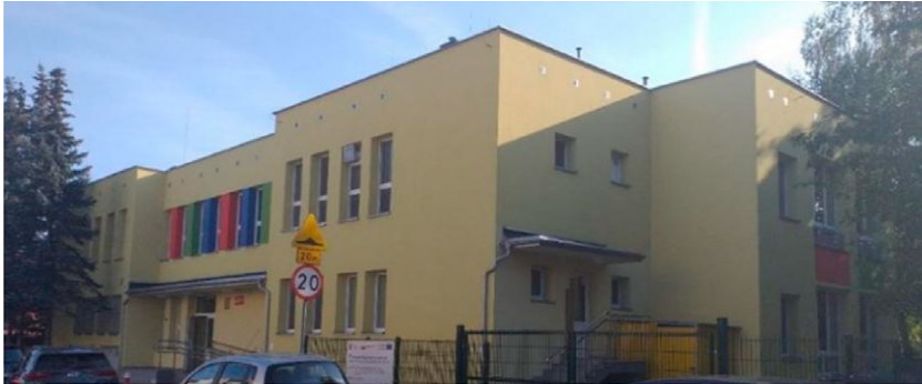
Figure 2. The view of the kindergarten building under consideration
