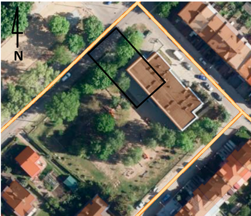
Figure 3. View of the location of the tested building with its layout on the plot
