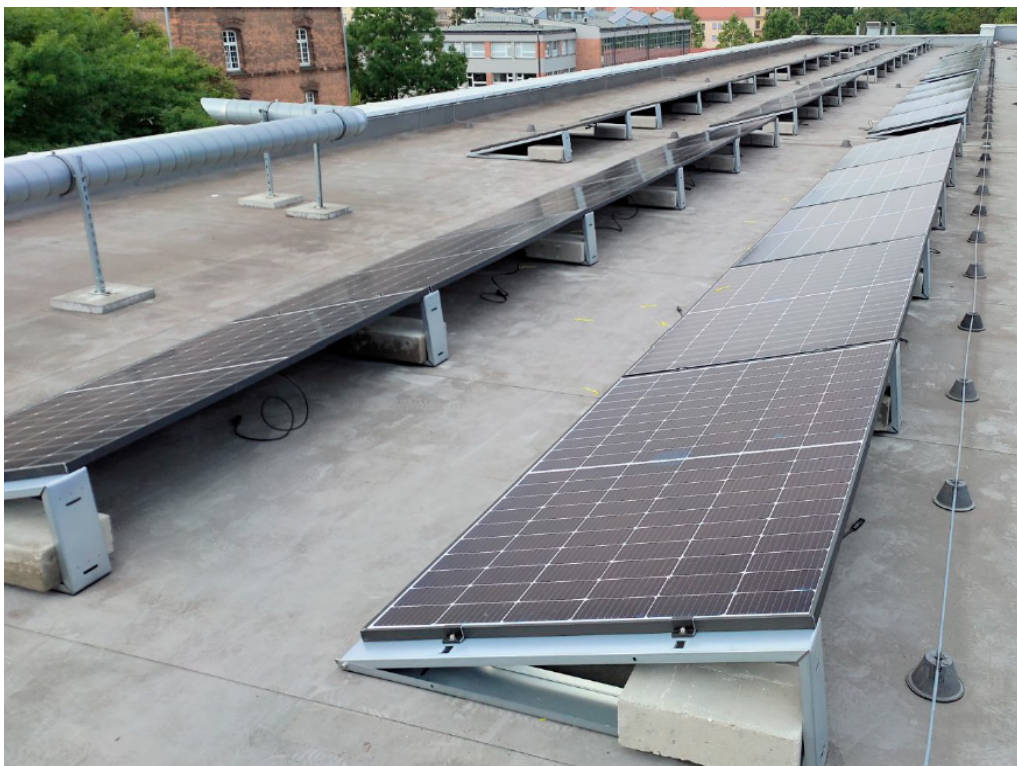
Figure 1. Panels of the photovoltaic system mounted on the large area flat roof with a non-invasive ballast system, without structural connection to the existing building bearing structure
