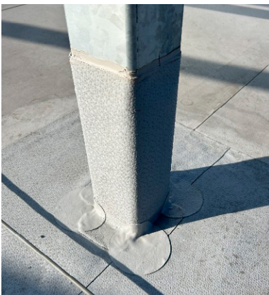
Figure 15. Roof covering treatment ensuring water-tightness of such covering in the area penetrated by the supporting column of a single photovoltaic system segment
